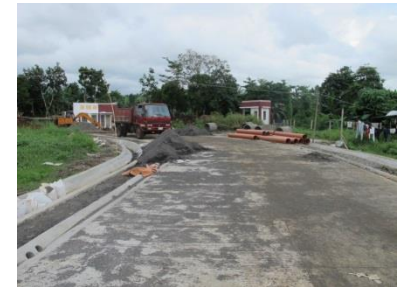
Construction of waste-water treatment facility
