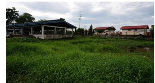
Slaughterhouse and existing wastewater ponds
